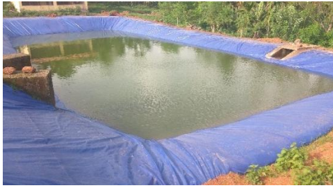
Small size pond ( V=300\text{ m}^3 D= 1.5\text{ m} )
